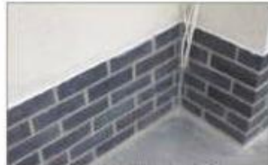
Face brickwork in dark grey-black semi engineering work
