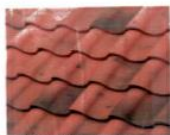
Clay pantiles on roof area of cart-lodge plot 4.
