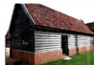
Red brickwork plinth with black timber weatherboarding over.
