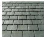
Natural slates to plot 4 main dwelling roof area and roof areas of cart-lodges serving plots 1 and 2.
