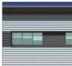
Aluminium curtain walling/ window system with internal structural box sections with polyester powder coat finish and double-glazed with anti-sun structural glazing units.
