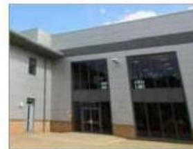
Aluminium curtain walling/ window system with internal structural box sections with polyester powder coat finish and double-glazed with anti-sun structural glazing units.
