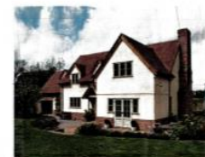
Red brickwork plinth with painted render over.
